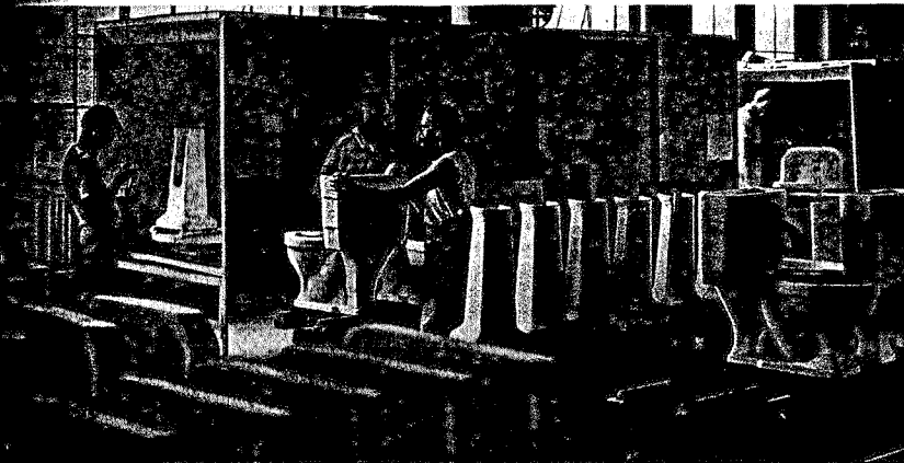
Applying color to Crane china plumbing fixtures with spray guns.
