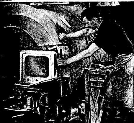
Huge grinding wheels smooth and finish the rims of Crane china fixtures.
