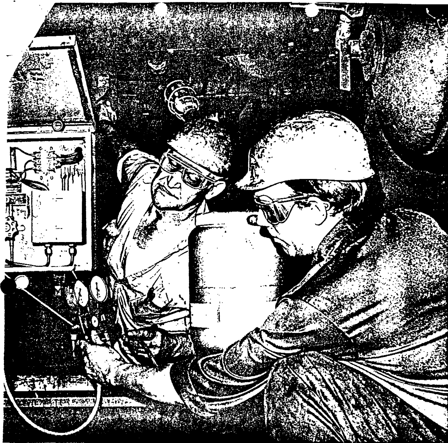
Sophisticated tools should be used in charging a system with refrigerant and checking for leaks.
