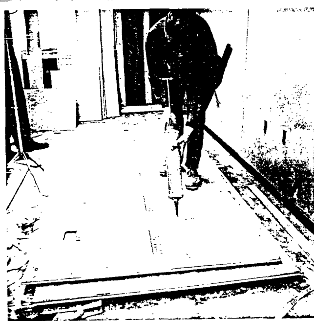
Applying Grabbit to Dens-Cote Base
