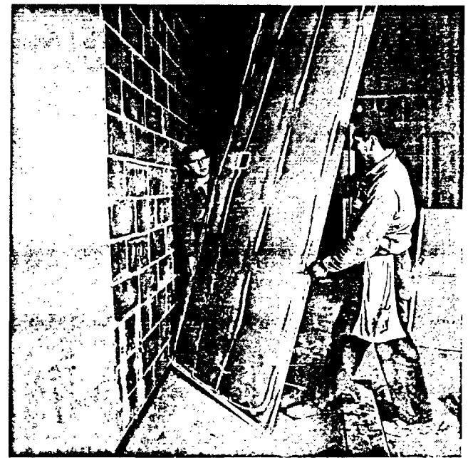
Installing Dens-Cote Base on Masonry Wall
