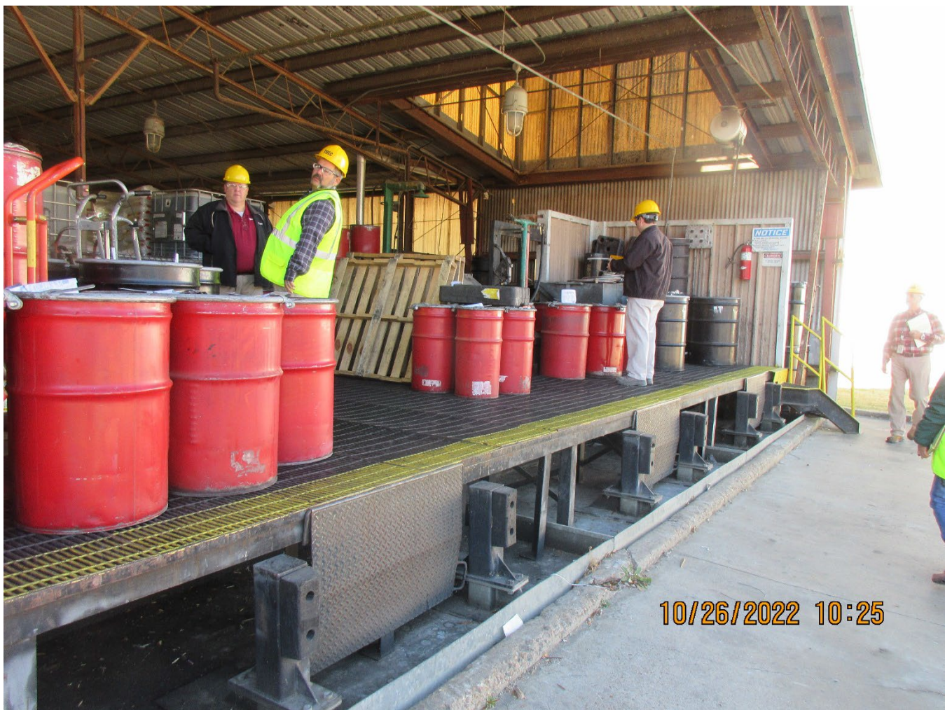
Photo 4 – Northwest Return and Fill Station
