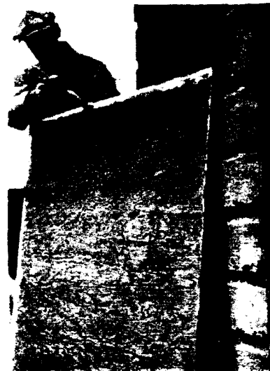
Specifications required that edges of all panels be primed with white lead before setting
