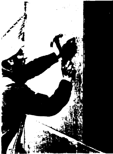
All panel edges were caulked with white lead paste and ship-lapped forming tile-like joint
