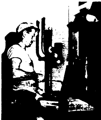
Wiping a joint in the lead waste line being installed in the offices of the Republic and Daily Herald, Yakima, Wash.
