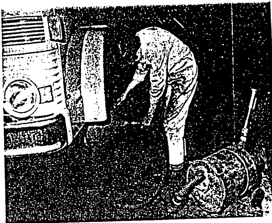
FIG. 1. Funnel method of dust control.
