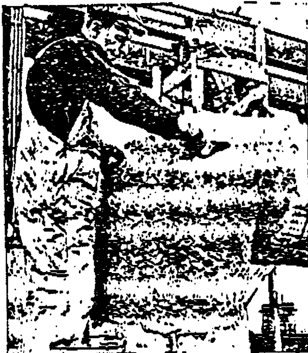
The workman is applying a coating of insulating cement, which adheres firmly to the wire netting. When dry, a weatherproof coat of O-C Mastic Finish will be applied.
