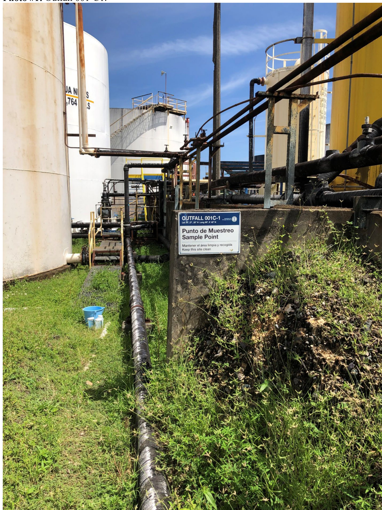
Photo #1: Outfall 001-C1.
