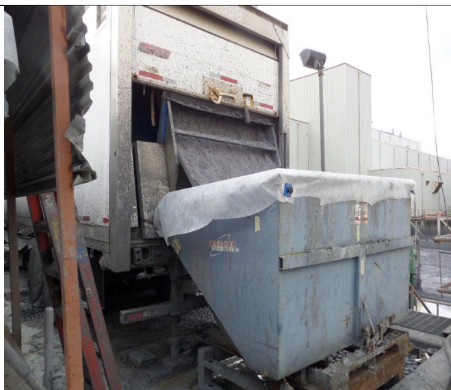
WWTP. Belt Press used to dewater solids. Observed waste solids in containment area. Photograph 6 taken at 10:49 a.m.
