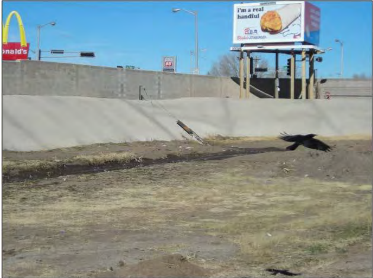
Photo Information: The outflow from the storm surge pond to the AMAFCA system.
