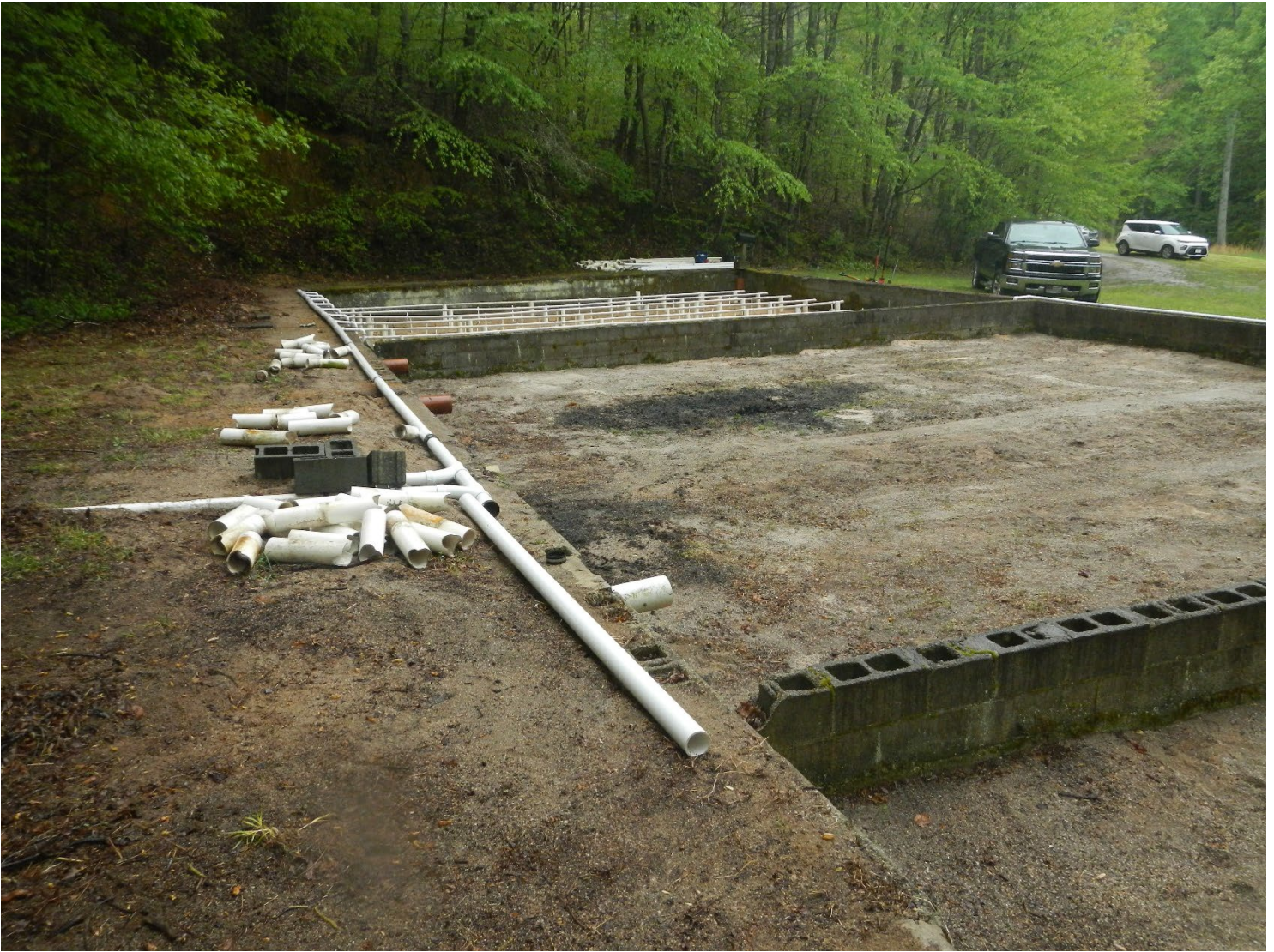
Figure 1 Sand filter system disassembled for repairs.
