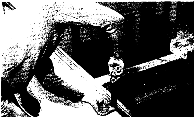
1. INSTALLING FLOOR TRACK.
