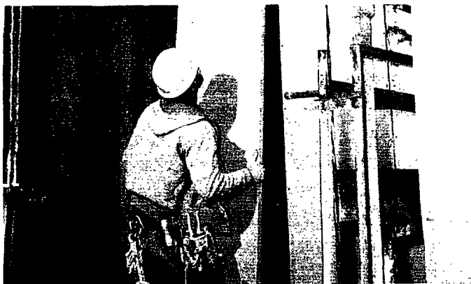
2. INSTALLING CORE PANEL.
