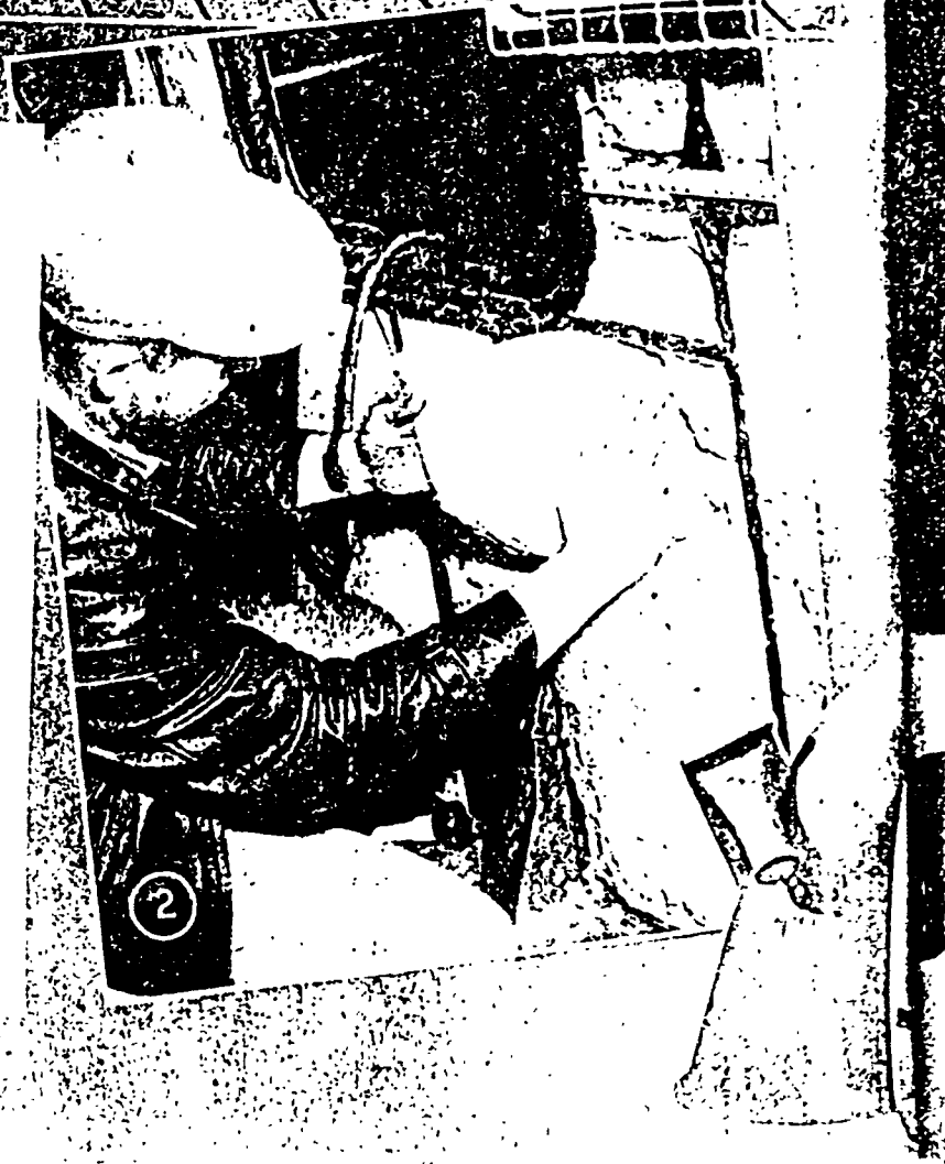
Fig. 1—Glass-fiber thermal insulation being installed in the roof of an industrial plant
