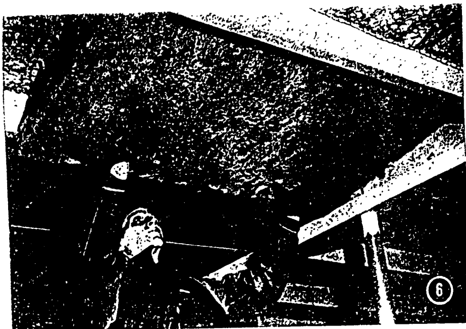
Fig. 6—Installing glass-fiber thermal insulation in the refrigerated compartment of a merchant ship
