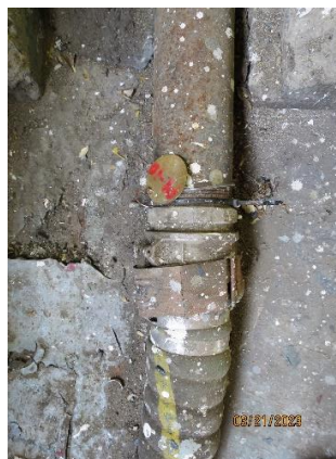
Photo #12 – Cracked floor in the containment of ancillary equipment.
