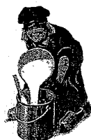
After giving it a quick stirring, pour the soft paste into a mixing bucket.
