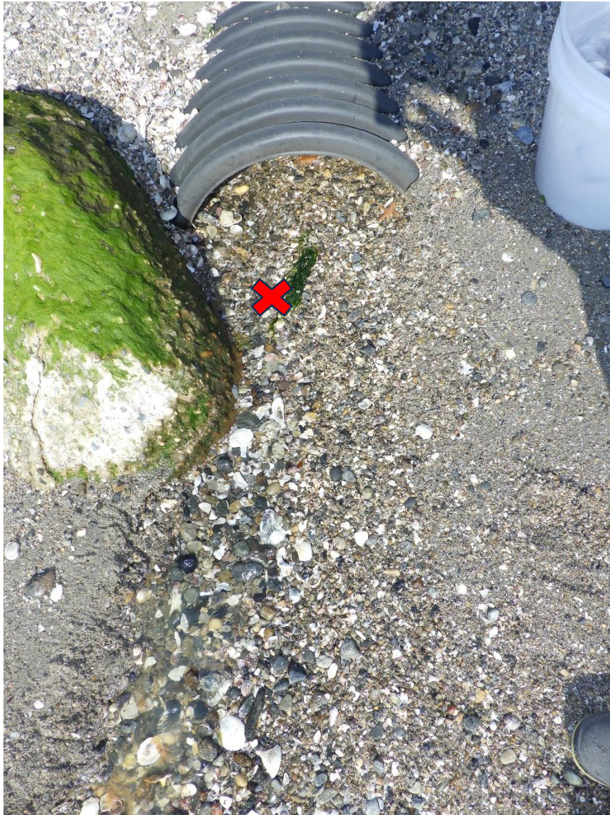
Photo 3: Seaside1 (photo taken 10/22/2024 at approx. 11:56) Outfall located adjacent to Seaside Park on Soundview Drive, discharging into Long Island Sound. Sample point is indicated by a red X.
