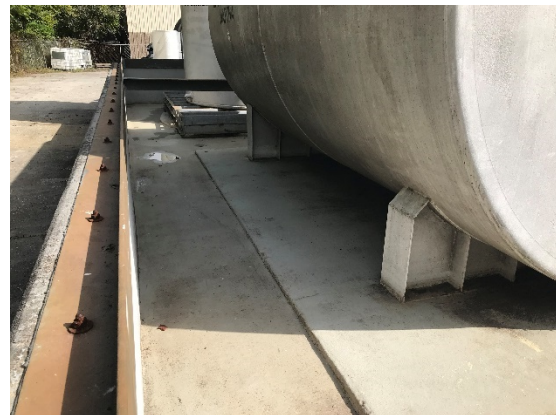
Picture 12: No Leaks and Spills in Secondary Containment of Hazardous Waste Tank #1
