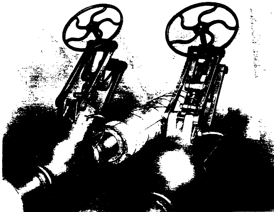
Special 12-inch 1500-Pound Crane Pressure-Seal Bonnet Globe Y-Pattern Stop Check Valves installed in the main steam lines of a central station operating at 900 pounds 900° F
