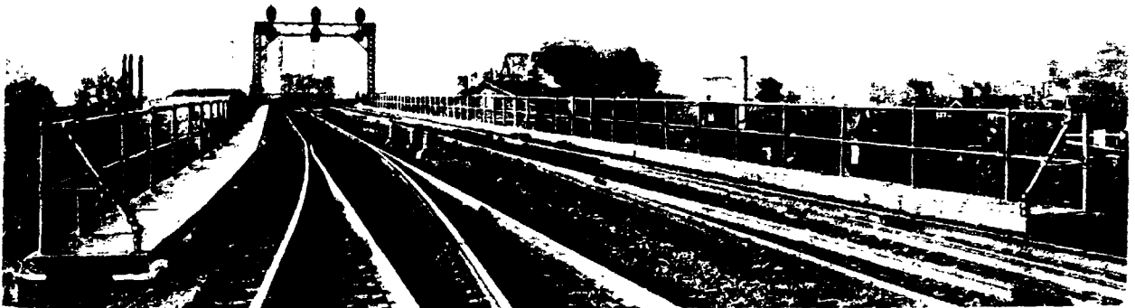
2-inch Galvanized Double Pipe Railing — total length of railing 6000 feet Fabricated in a Crane Branch House Shop
