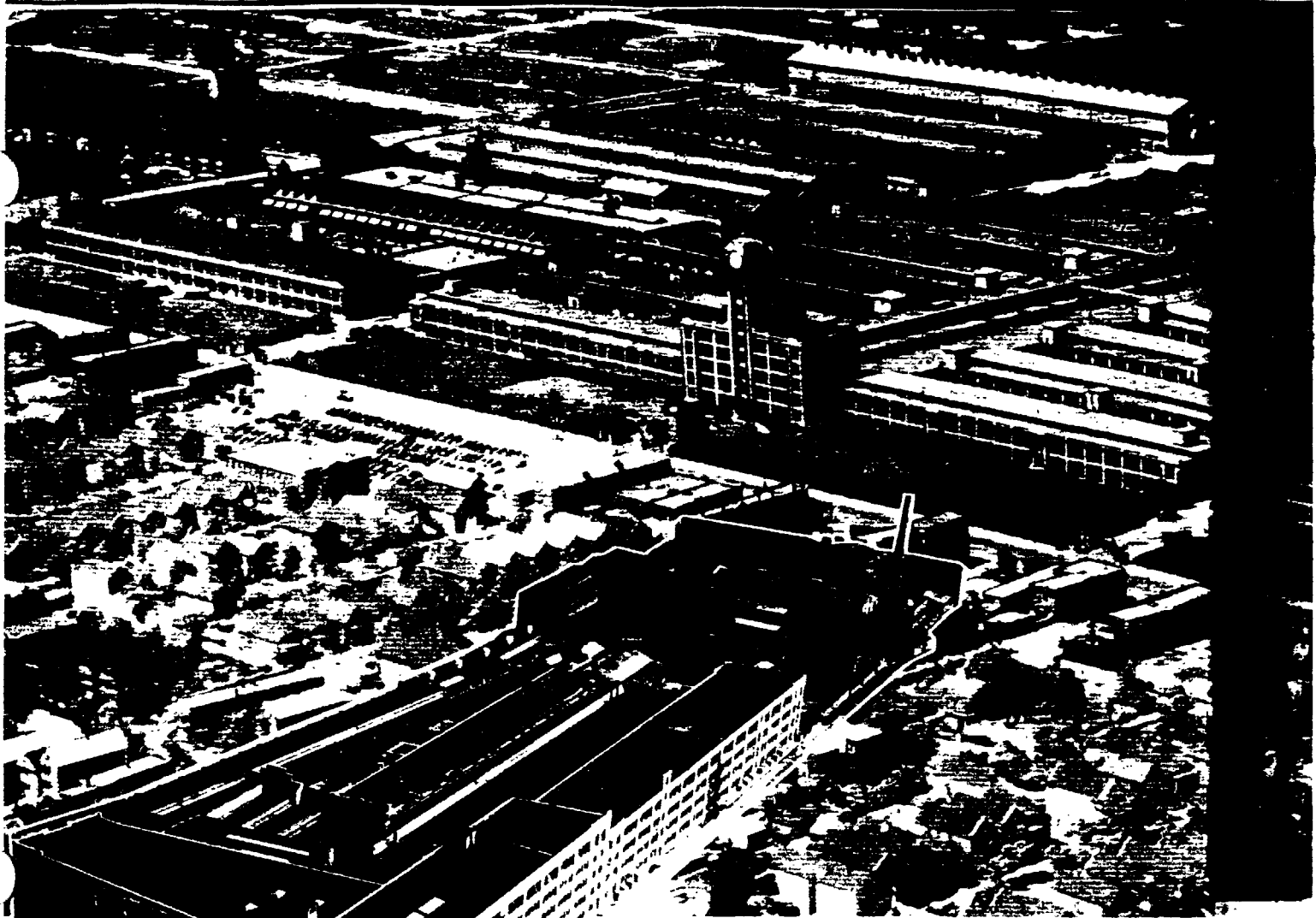
(Left) One of the two Crane Plants at Trenton, N. J. (Trenton Potteries Co.)
