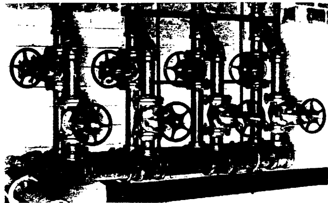
Crane valves in cooler lines of a brewery.
