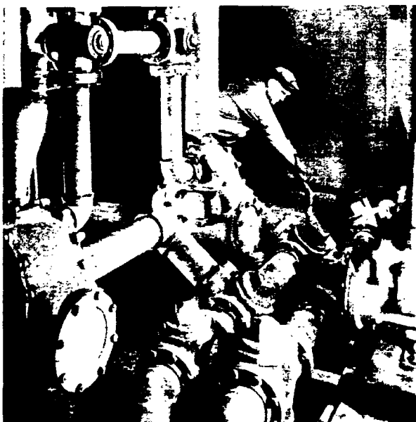
Crane Cocks in an intricate pumping system.
