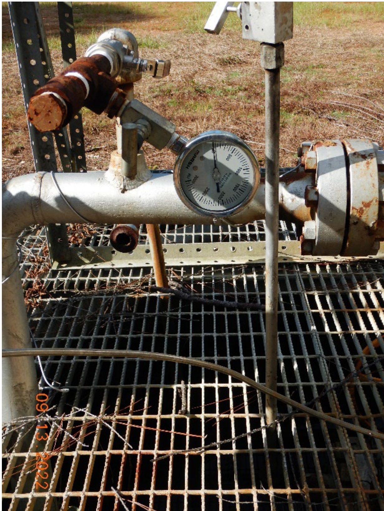
Photograph 4: Looking south, closeup view of production casing pressure gauge reading 0 psi.
