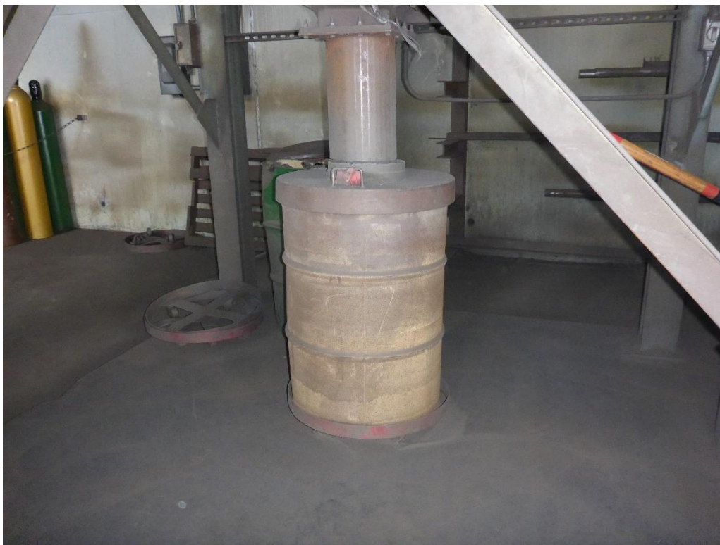
Photo 19: 55-gallon drum under Wheelabrator Baghouse. The drum is not labeled.
