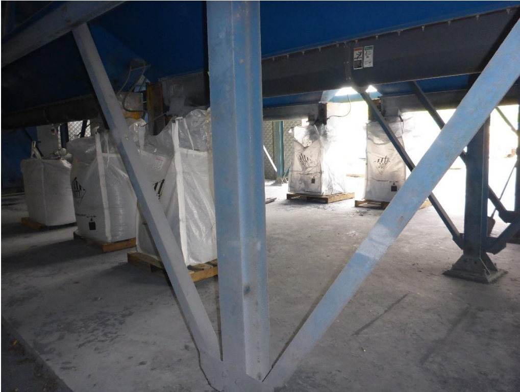
Photo 29: Four supersacks observed connected to the Furnace Baghouse. Additional supersacks stored in this area. Bags identified with DOT class 9 hazard placard, but not labeled. Personnel stated that the bags contain furnace ash, which is sold as zinc.
