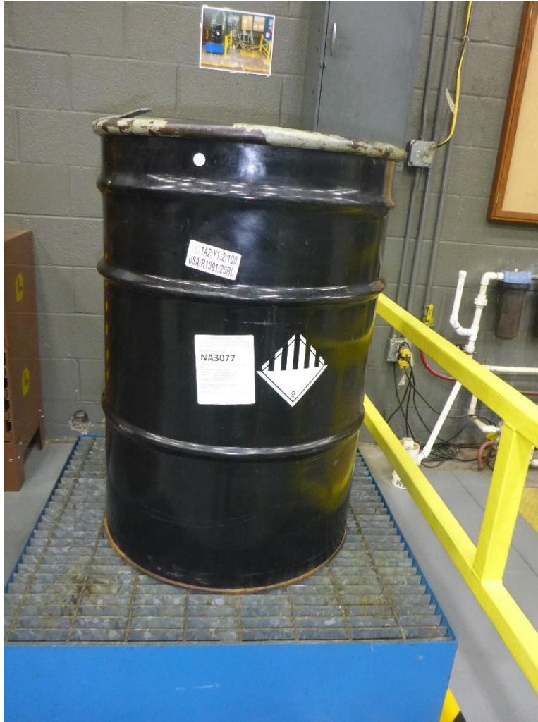
Photo 25: SAA for accumulating mop heads and used filters generated in the filter system for the hand sinks. 55-gallon drum labeled D008 hazardous waste contaminated debris and identified with a DOT class 9 hazard placard.
