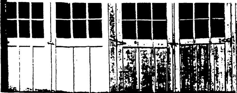
The two source doors to the left are in SWP House Paint and the two to the right in lead and oil. This un-retouched photo shows why your customer likes SWP service. Observe how the windows have rotted through the white lead. This 2 1/2 year old job tells a story better than words.
