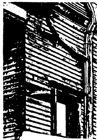
An extreme case—rotted in work—made rotten determining siding to fall out.
