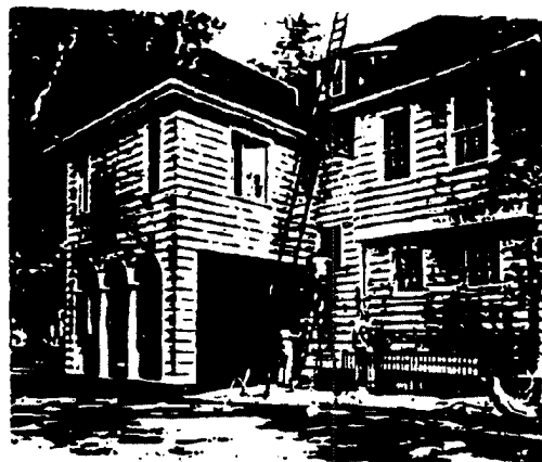
This house in Massachusetts shows the results of excellent maintenance as well as good paint. SWP had protected the surface well and was in good condition for re-paint after 18 years exposure.
