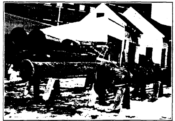
LEFT Cast iron pipe line with lead joints laid in 1854 at Nashua, N. H.
