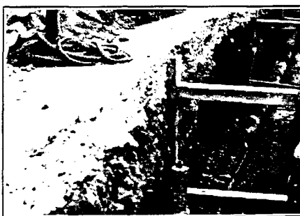
LEFT Cast iron pipe line with lead joints laid in 1854 at Nashua, N. H.
