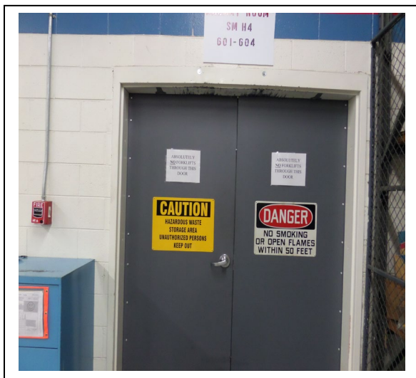
SAATI. 90-Day or Less Accumulation Area. Inspectors observed signs identifying the storage area. Photograph 9 taken at 11:49 a.m.
