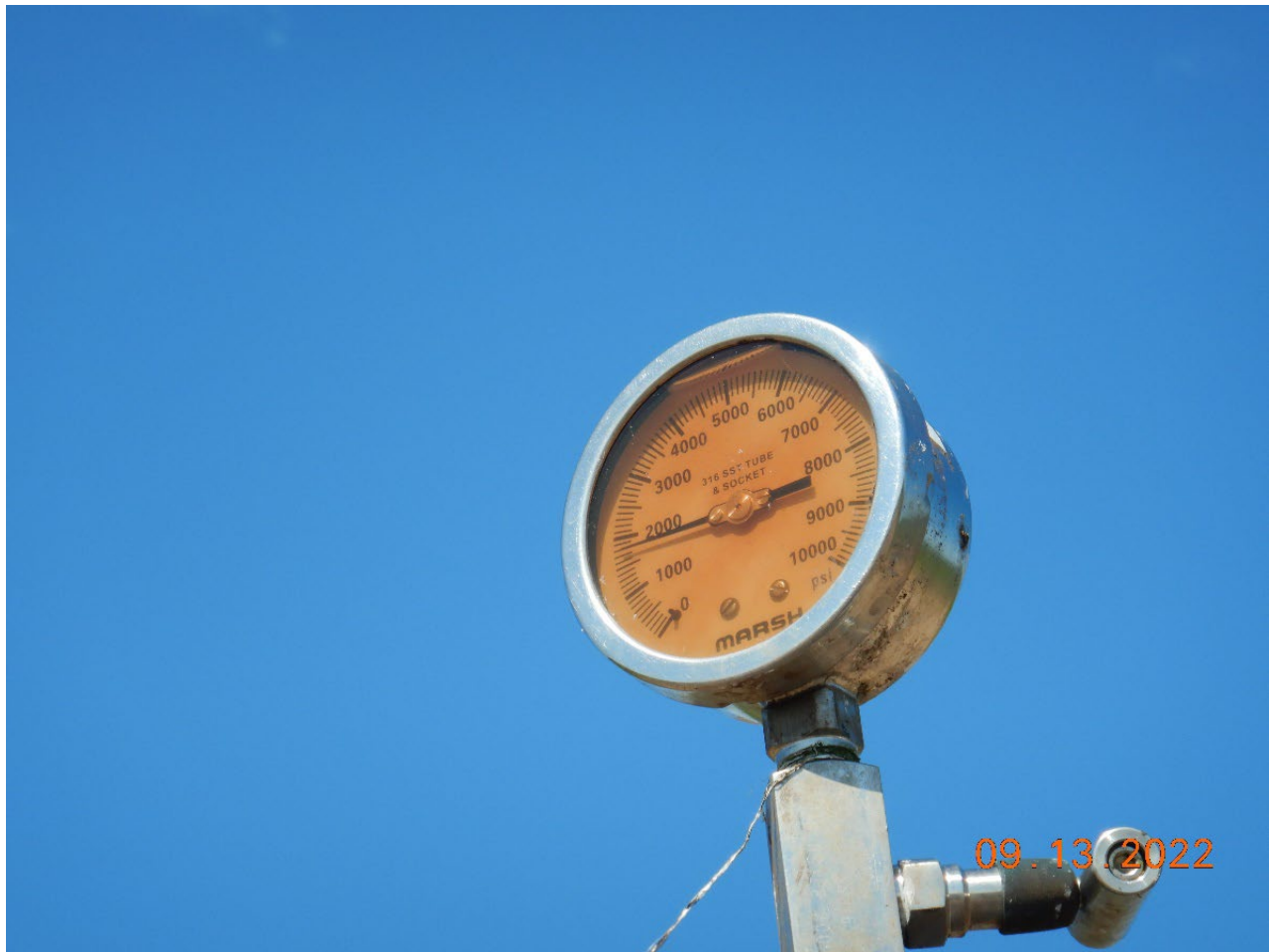
Photograph 6: Looking west, view of internal pressure gauge reading 1,750 psi.
