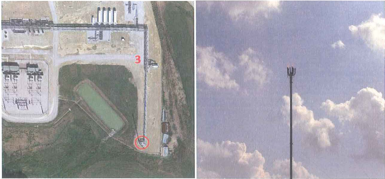
Figure 3. High Pressure (HP) Flare. Left: Google map with a red circle indicating the location of the flare and a red number “3” indicating the location of the VISR instrument. Distance: 369 ft. Right: A photo of the flare taken during the test.
