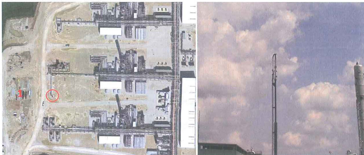
Figure 1. Tank Flare. Left: Google map with a red circle indicating the location of the flare and a red number "1" indicating the location of the VISR instrument. Distance: 150 ft. Right: A photo of the flare taken during the test.
