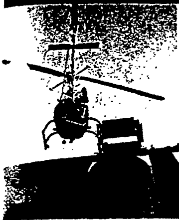
Helicopters were used to transport some of the assembled units for the Oroville Dam project.
