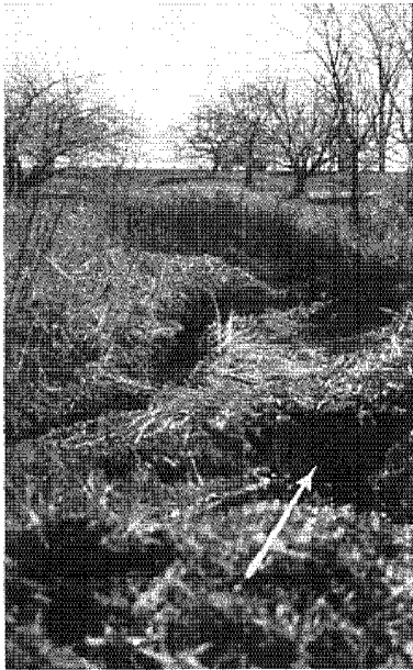
Above—The arrow shows point where ten-inch tile culvert crosses under highway. Right—Stumps blasted but not removed
