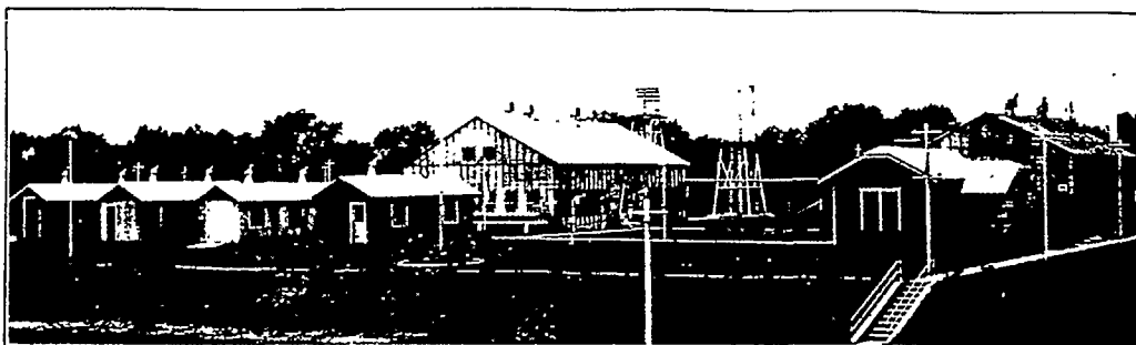
(Above) This station of the Oklahoma Natural Gas Company at Owosso, Okla., is thoroughly modern in every respect. Swartwout Ventilators help to make it so.
