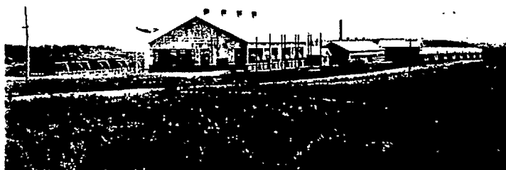
(Left) One of many Cities Service Gas Compressor Stations, Swartwout equipped.
