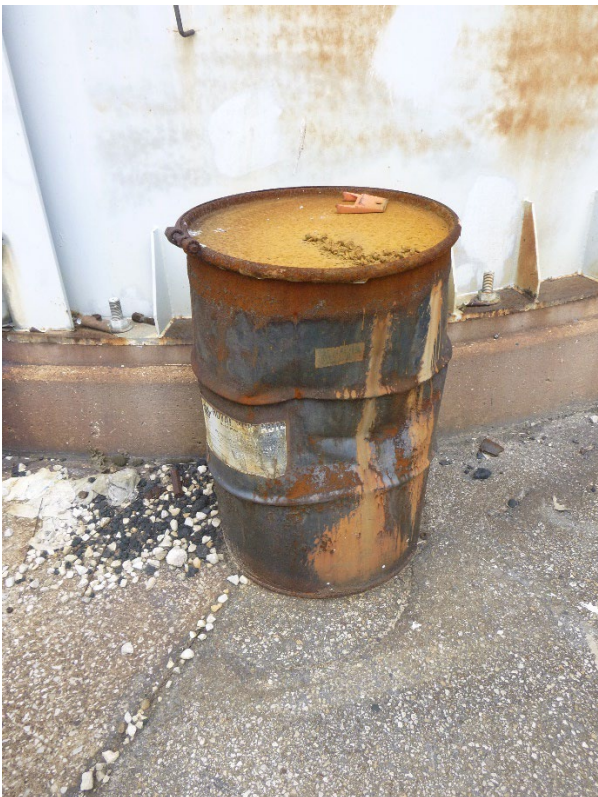
Photograph 13: Unknown contents in container at base of scrubber tower.
