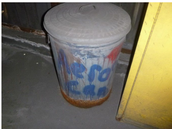
Photograph 6: Rodding Department SAA for spent aerosol cans – no hazardous waste liable or indication of hazard.
