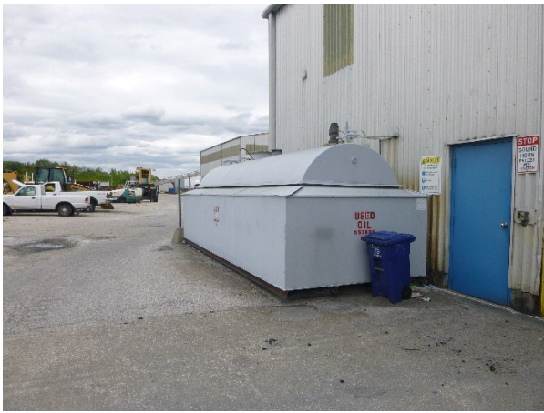
Photograph 33: Mobile Garage Used Oil Tank.
