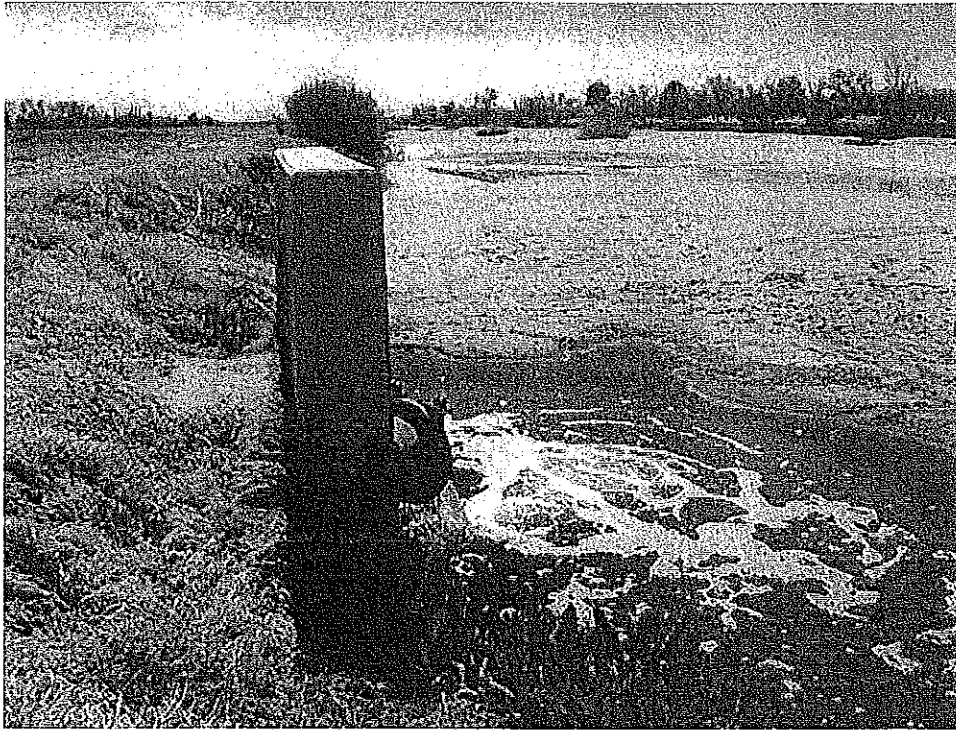
DP-450 Anthony discharge to Rio Grande 03-09-16; Looking downstream
