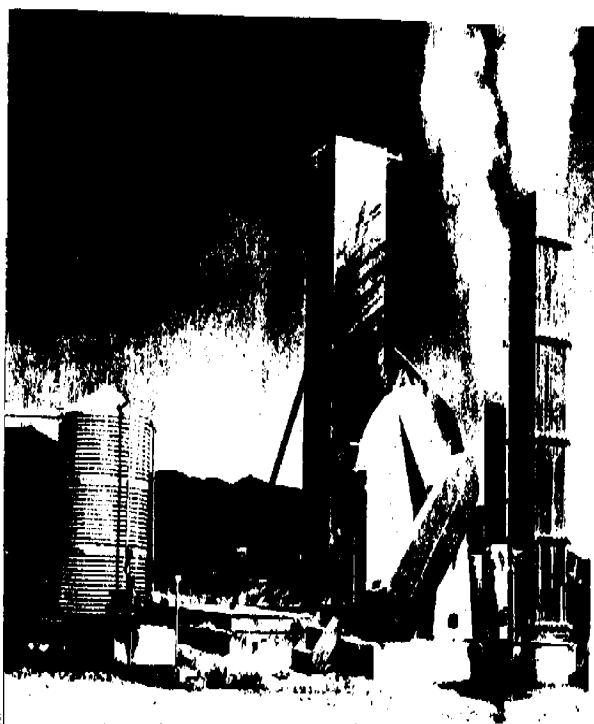
A Roto-Clone, part of the system of wet dust collectors which is one of the most important accomplishments in J-M's extensive program to control dust throughout its operations. Fine residual particles of diatomite contained in combustion gases and steam from processing are here removed from the vapors as they pass through a curtain of water. Heavier particles are first removed by settling in a huge chamber excavated in the hill beneath the Roto-Clone.
