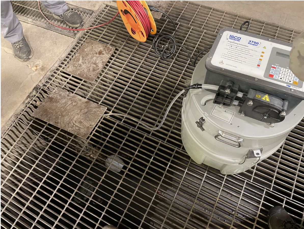
Figure 1: Outfall 001 Composite Sampler Set-up Taken 7/18/23 10:23 am
