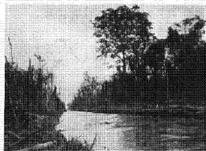
A closer view of the finished ditch a little farther up the line
