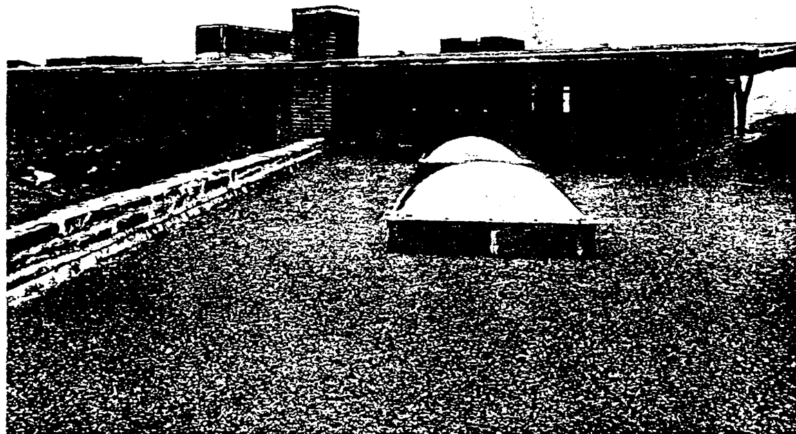
Lead flashings on the skydomes and walls, lead chimney caps, and a lead facing strip and gravel stop around the roof are features of this ultra modern home in Randolph, Vt. See story page 2.
