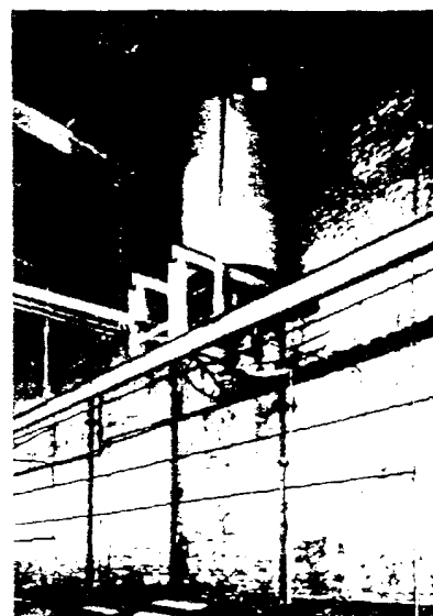
Detroit Sulphite Pulp and Paper Company's 500 gal. lead-lined liquid alum auxiliary storage tank.
