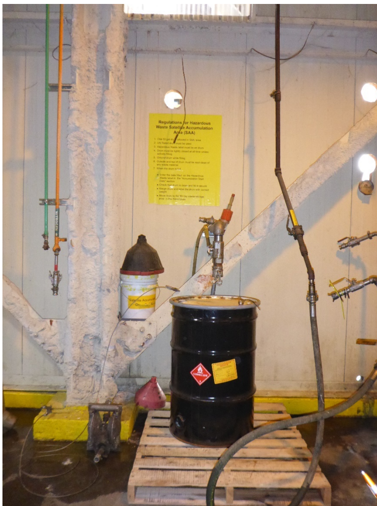
Photo 2: One 55-gallon drum located in the West Plant SAA. The drum was closed, labeled D001 / F003 hazardous waste flammable liquid (methanol / ethanol) cleaning alcohols, and identified with a flammable liquid DOT hazard placard.
