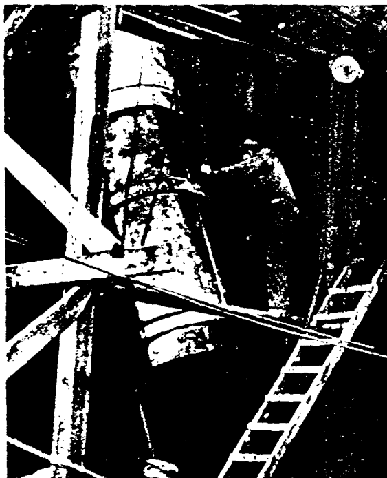
Below, preparing to remove the mandrel from a completed section of the lead duct. Note that steel struts which provide both stiffening and support are secured to the duct and sealed off from corrosive atmosphere by sheet lead covering burned to the duct wall.
