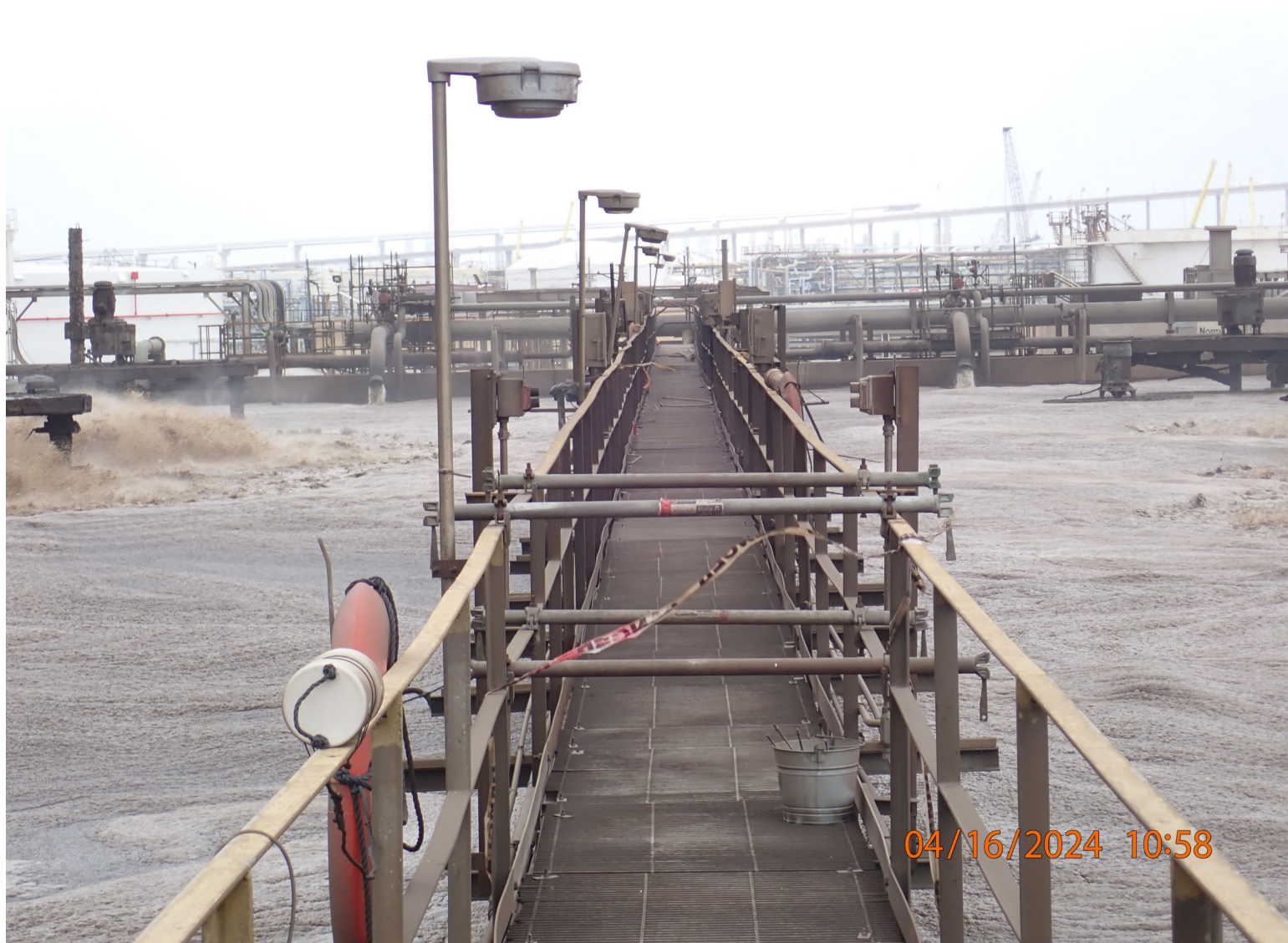
Photo 003: NET Aeration Basin, North and South "Pour" Inlets 4/16/2024 09:58 P4160003.jpg
