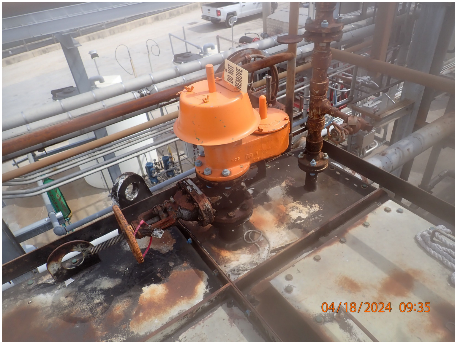
Photo 022: CPI #2 Vacuum Breaker - 4/18/2024 P4180022.jpg
