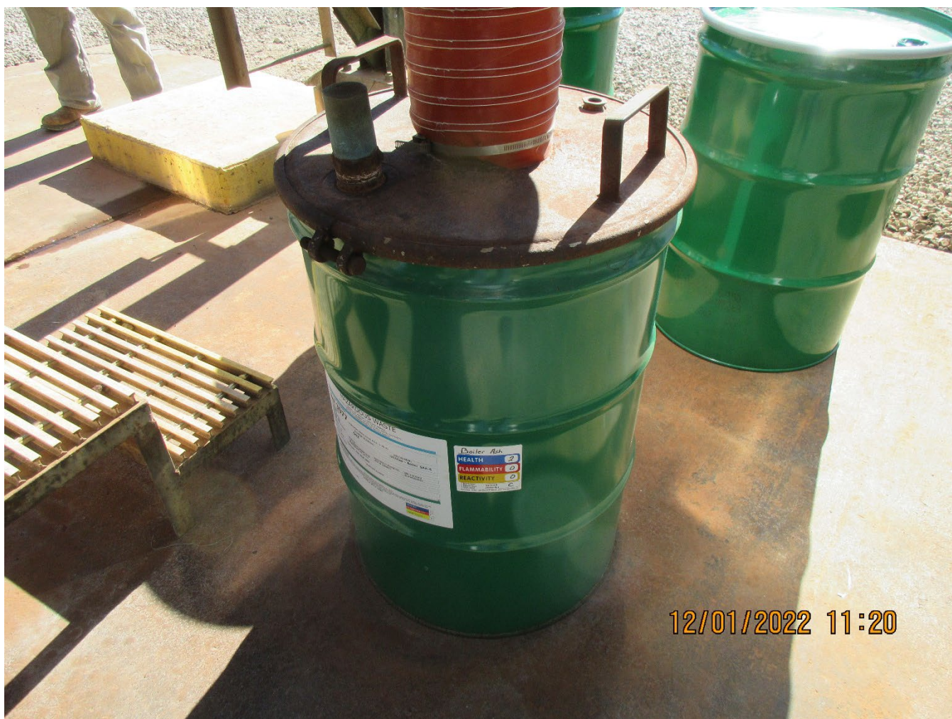
Photograph 6 – Container for ash from Boiler #4's Baghouse
