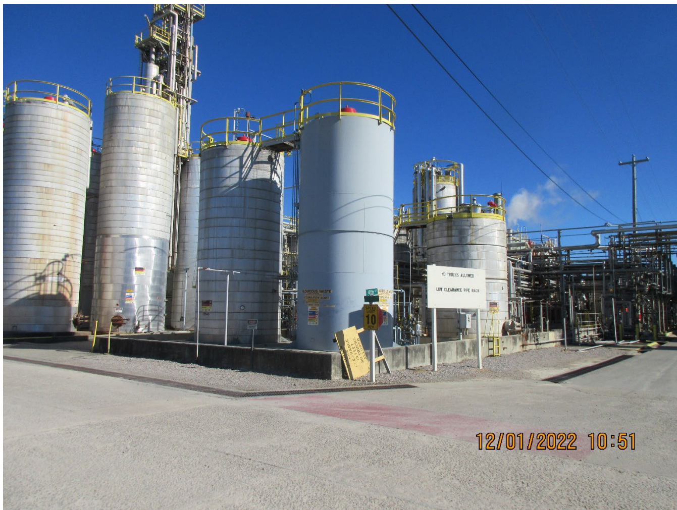
Photograph 1 – Tank 8155 (center foreground)
