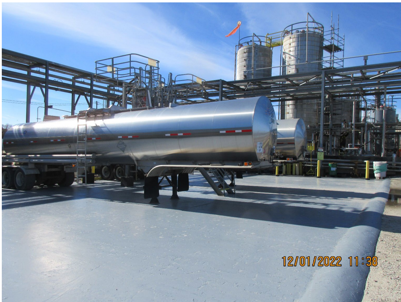
Photograph 9 – Tanker Trailer Pad
