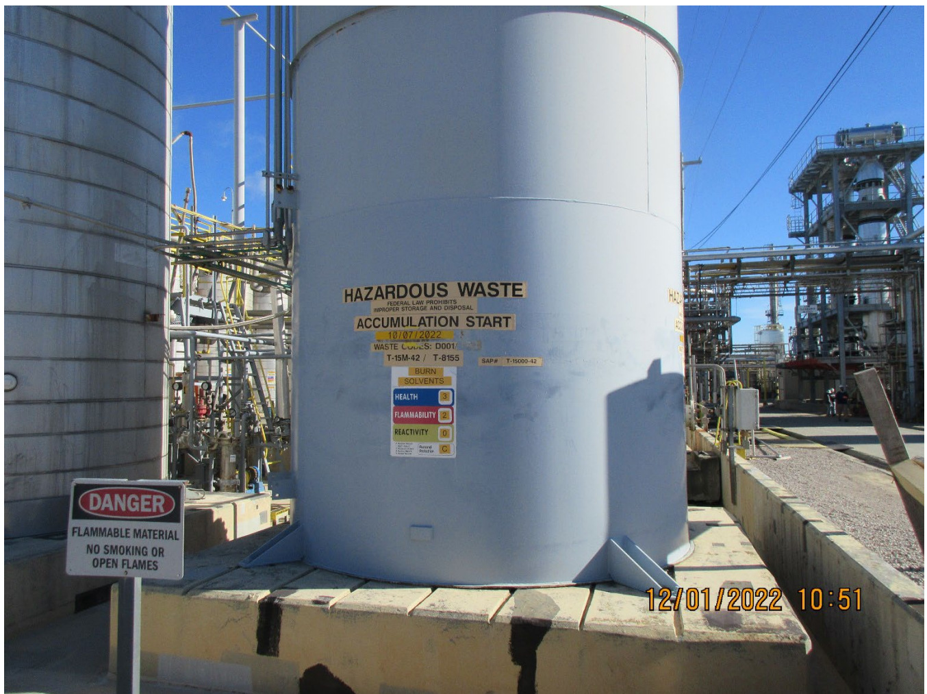
Photograph 2 – Labeling on Tank 8155
