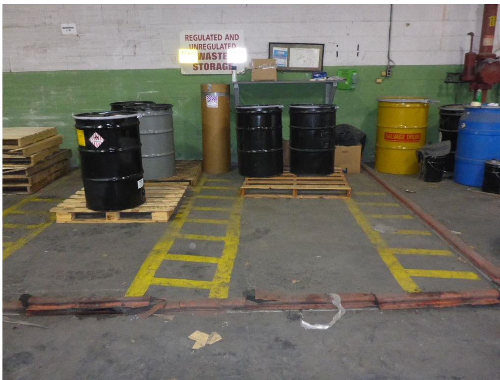
Photo 14: Main hazardous waste central accumulation area. Several gaps in the secondary containment berm around the perimeter of the area.
