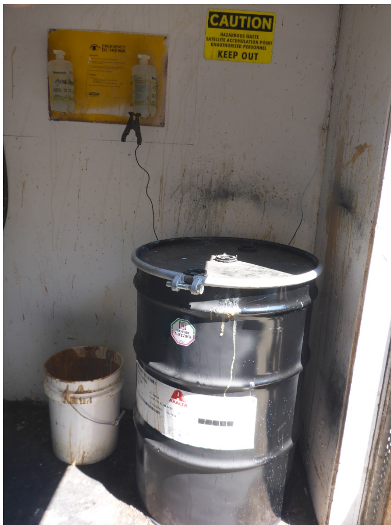
Photo 3: Wood Plant SAA for accumulating hazardous waste silt bottoms in the distillery. 55-gallon drum was grounded and closed, and reported to be empty.
