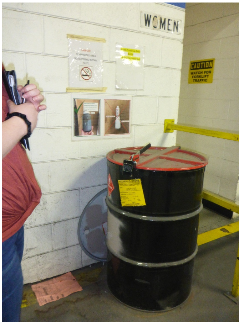
Photo 13: SAA for accumulating waste touch-up paint bottles in the Metal Plant. 55-gallon drum with latched flip-top lid labeled D001 / F003 / F005 hazardous waste loose flammable containers.
