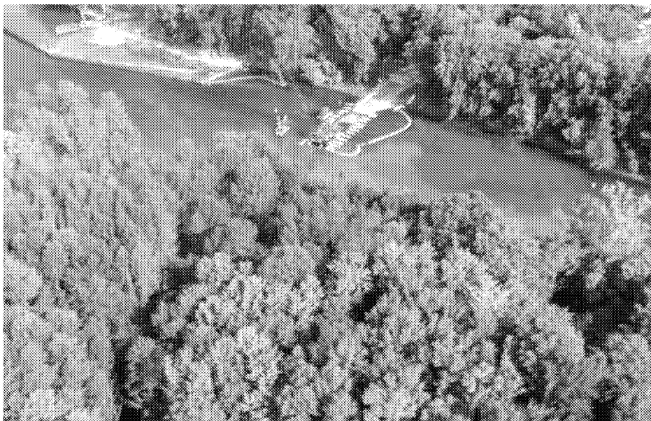
In-channel sediment removal
