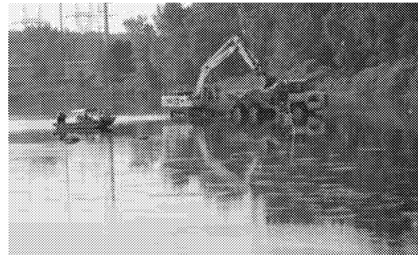
Installing armor stone over the sediment management area in SMA 1-5.
