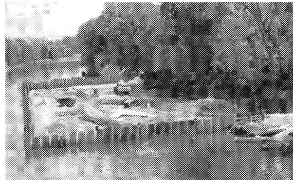
Removal of river sediment with direct loading into trucks for transportation and disposal.
