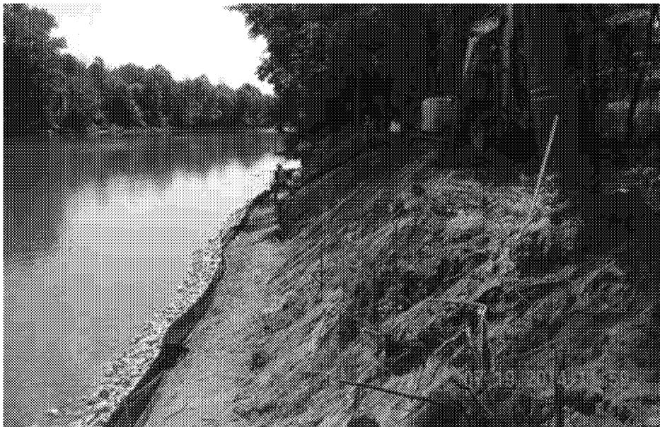
Bank preparation for stabilization including canopy management
