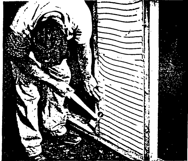
E. Position sidewall blocks between studs and hold flush with face by wallboard strips which have been recessed against sides of studs. Blocking must be flush or slightly behind nailing face of studs.
