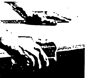
Smooth cut edges with a rasp, coarse sandpaper or metal lath wrapped around a block of wood, or trim with a cutting knife.
