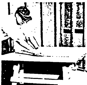
Score paper on face of board with cutting knife, using a straight edge as a guide.
