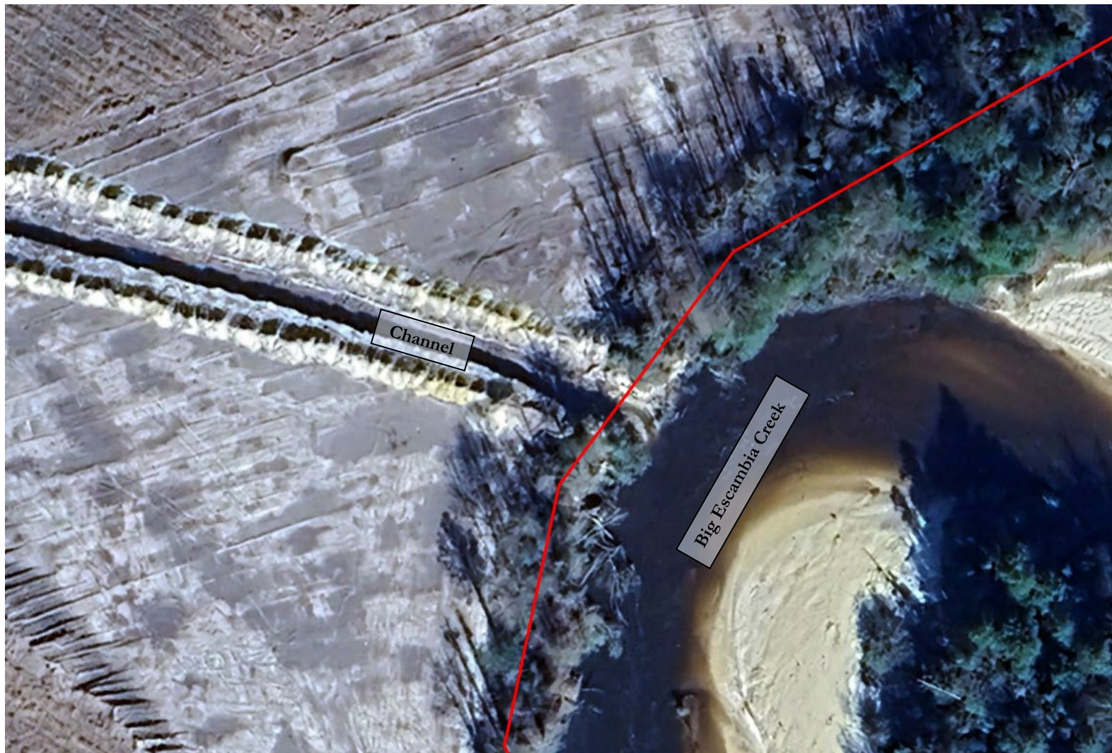
Figure 5. GoogleEarth aerial image showing close-up of excavated channel from Figure 4 and its confluence with Big Escambia Creek, imagery dated January 13, 2023. The red lines indicate the approximate Facility boundary. Also refer to Appendix B, Photographs 8 through 11.
