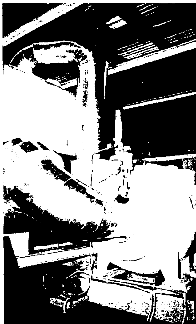
Verne Traudt inspects 5200-ton Chiller-Compressor #3 at the city power plant (left). Chiller #4 is seen (right), as well as compressor, and freon discharge line.
