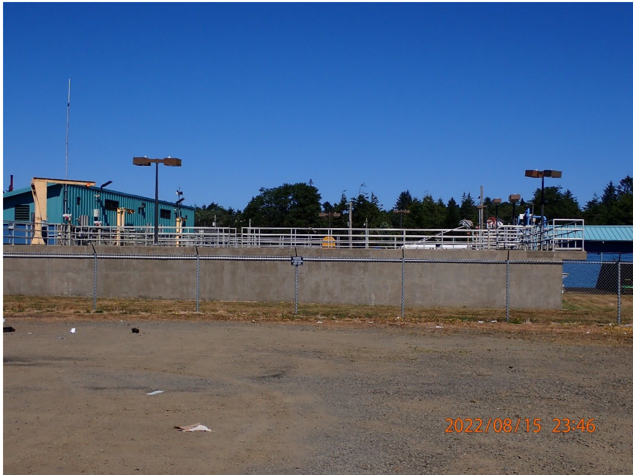
Photo 11 - City of Ilwaco WWTP
