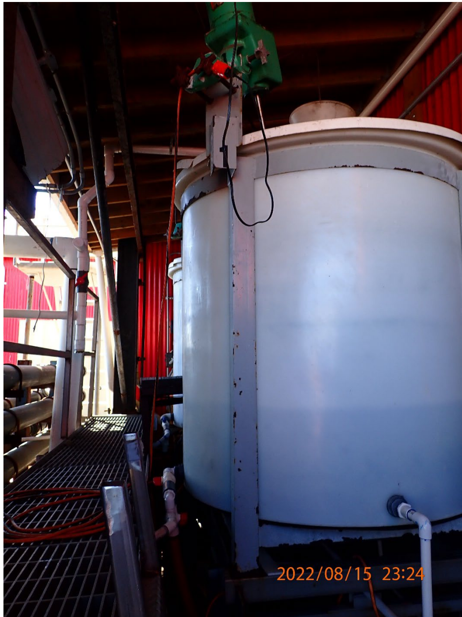
Photo 7 - Flocculation Tanks
