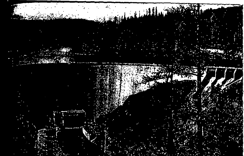
ALDER DAM and powerhouse form largest single unit in Nisqually No. 2 development. The dam, a variable-radius concrete structure, 330 ft high, 1500 ft long, 120 ft thick at base, forms a storage reservoir of 210,000 acre-ft capacity.
