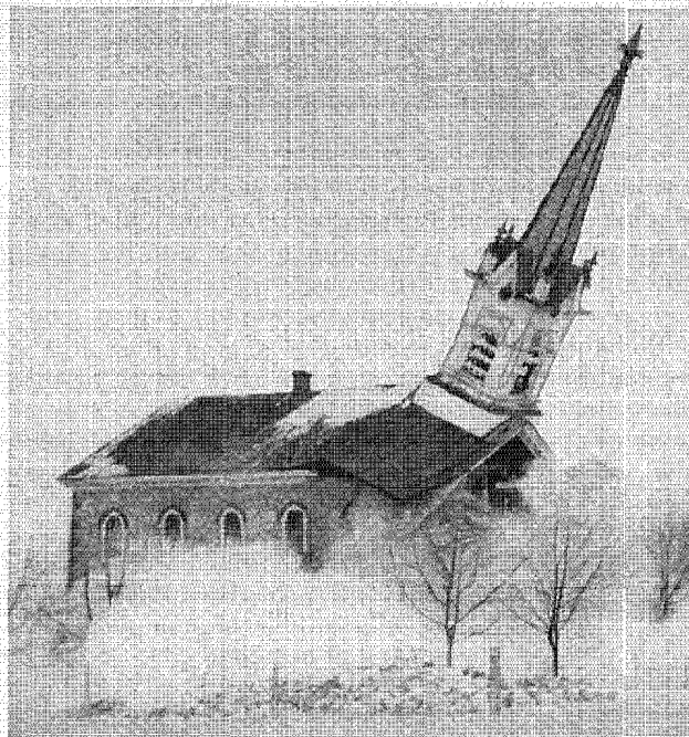
At the moment of the blast. A few seconds later the entire structure was only a broken mass of stone and wood and twisted tin.
