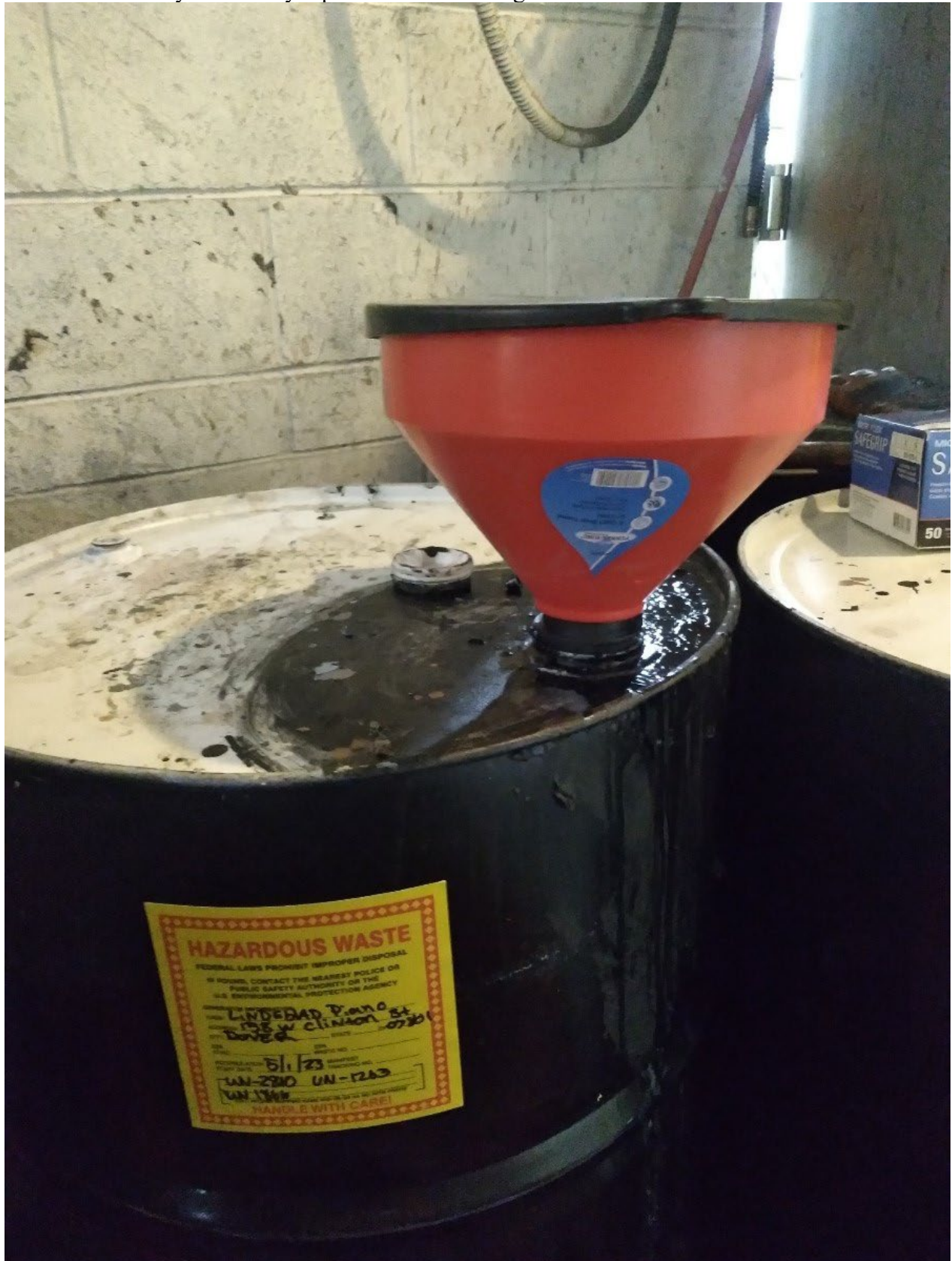
Photo #4: Sent by the facility representative showing closed funnel and hazardous waste label.
