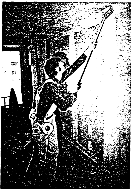
Figure 1 — Pole sanding of drywall taping compounds. Several applications of taping compounds may be required to make a smooth join between gypsum wall boards, requiring extensive sanding.
