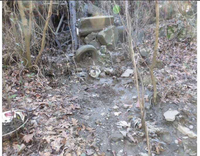
Wooded Area Behind Keebler North Bunker Area (see photograph 16). The inspectors observed a washout containing ASR material flowing from the outfall #3 pipe to ground surfaces. The inspectors took a split sample in this area. Photograph 54 taken at 3:21 p.m.
