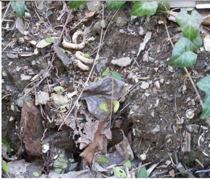
Keebler North Concrete Conveyance for Outfall #3. The inspectors observed ASR material accumulating on soil surfaces. Photograph 49 taken at 3:00 p.m.
