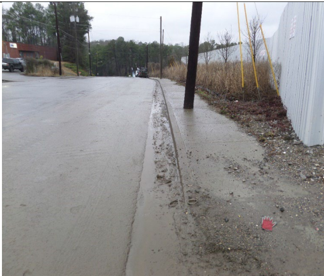
3320 Empire Boulevard. The inspectors observed ASR material on the east side of the road and north down the hill. Photograph 11 taken at 9:30 a.m.
