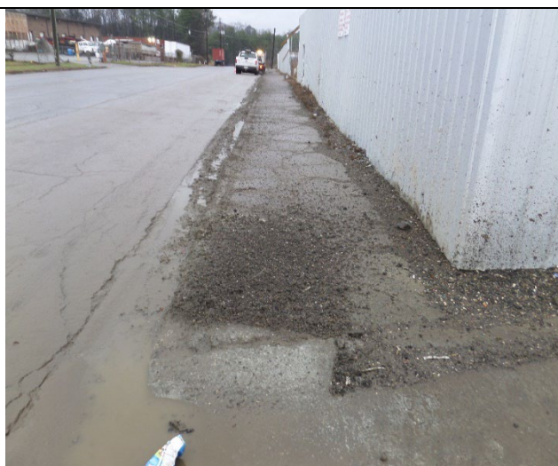
3320 Empire Boulevard. The inspectors observed the release of ASR material was from the 3320 Empire Boulevard south gate entrance. Photograph 6 taken at 9:30 a.m.
