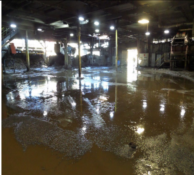
Keebler Plant Building Filter Press Area. The inspectors observed filter cake generated from the filter press accumulating with wastewater and solids on the concrete floor. Photograph 40 taken at 2:08 p.m.
