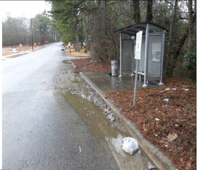
3320 Empire Boulevard. MARTA Bus Stop #178. The inspectors observed ASR material on the east side of the road and north down the hill to the MARTA bus stop #178 near South Industrial Park. Photograph 14 taken at 10:50 a.m.
