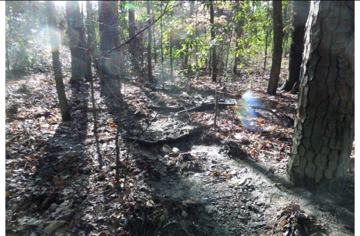
Wooded Area behind Keebler North Bunker Area. The inspectors observed a washout containing ASR material flowing from outfall #3 pipe downhill to the earthen access path. Distance from Outfall #3 pipe approximately 90-105 feet. General impression of Photograph 21. Photograph 22 taken at 11:30 a.m.
