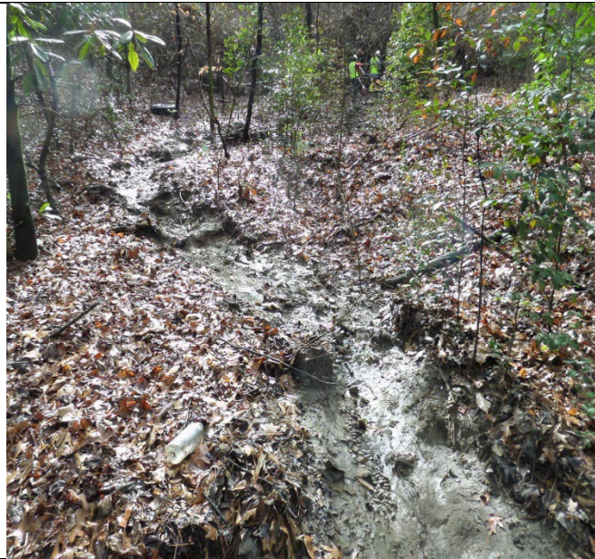
Wooded Area behind Keebler North Bunker Area. The inspectors observed a washout containing ASR material flowing from outfall #3 pipe to the earthen access path. Distance from Outfall #3 pipe is approximately 30-45 feet. Photograph 17 taken at 11:19 a.m.
