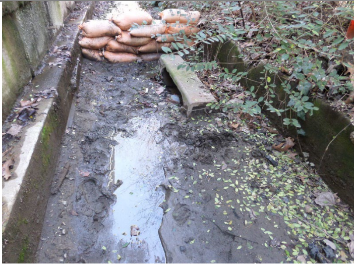
Keebler North Concrete Conveyance for Outfall #3. The inspectors observed a drain that discharges to the outfall pipe in the wooded area in Photograph 16. Photograph 47 taken at 2:59 p.m.
