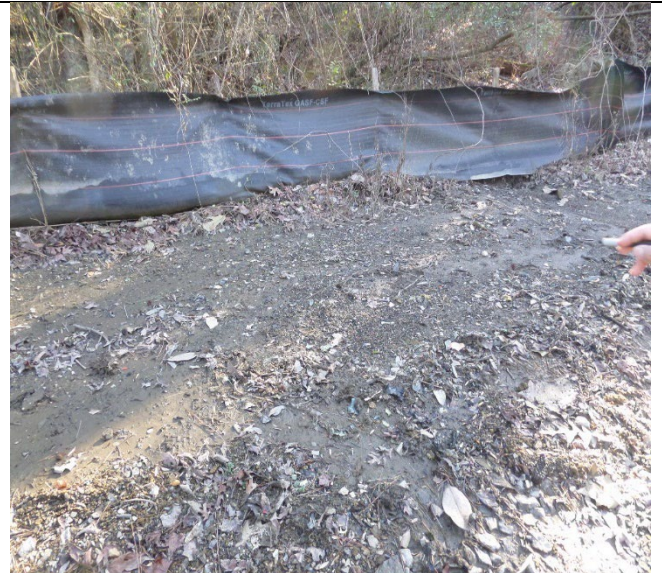
Access Path Next to Wooded Area Behind Keebler North Bunker Area. The inspectors observed a washout containing ASR material flowing from Outfall #3 pipe to the earthen access path. Distance from Outfall #3 pipe approximately 150-180 feet. Photograph 52 taken at 3:12 p.m.
