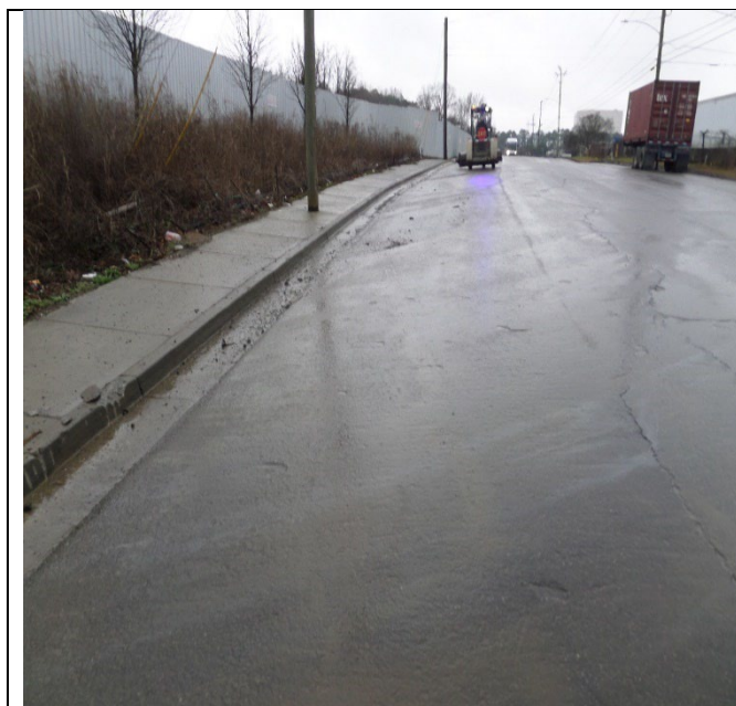
3320 Empire Boulevard. The inspectors observed ASR material on the east side of the road and north down the hill Photograph 1 taken at 9:30 a.m.
