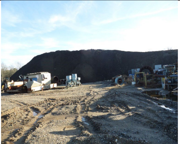
3320 Empire Boulevard ASR Pile. The inspectors observed a large ASR pile. Photograph 56 taken at 4:30 p.m.
