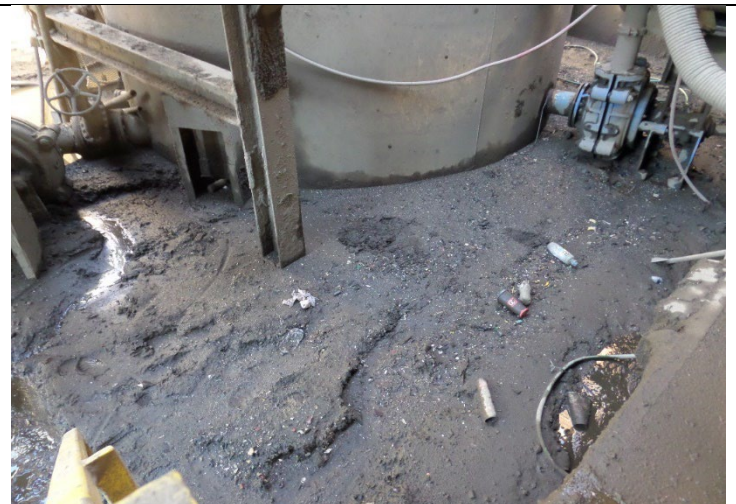
Wastewater Treatment Area. The inspectors observed solids/sludge containing ASR material accumulating in this area. Photograph 36 taken at 2:06 p.m.
