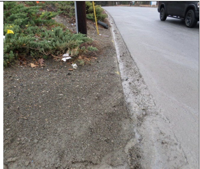
3320 Empire Boulevard. The inspectors observed ASR material on the ground along the edge of the driveway to 3311 Empire Boulevard. Photograph 12 taken at 9:38 a.m.
