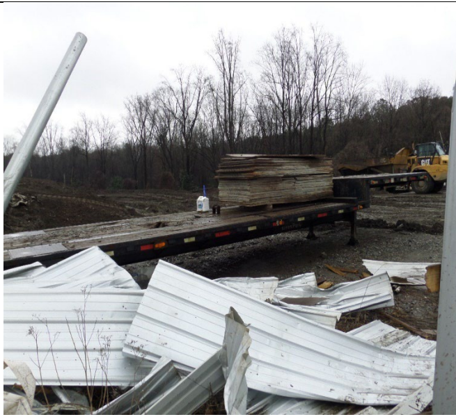
3320 Empire Boulevard. The inspectors observed ASR material on the east side of the road and north down the hill. Photograph 9 taken at 9:30 a.m.
