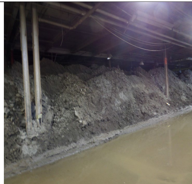
Keebler Plant Building Filter Cake Pile. The inspectors observed wastewater and solids accumulating on the concrete floor next to the Pile. Photograph 44 taken at 2:30 p.m.
