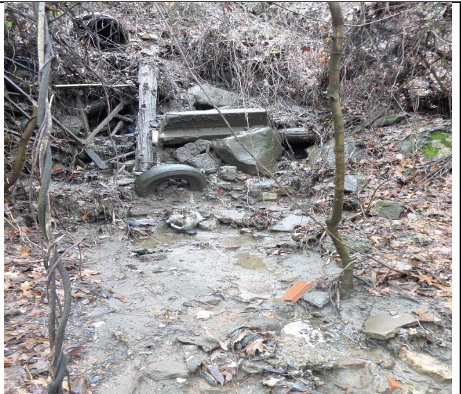
Wooded Area Behind Keebler North Bunker Area. The inspectors observed a washout containing ASR material flowing from the outfall #3 pipe to ground surfaces. See outfall pipe in top left corner of photograph. Photograph 16 taken at 11:17 a.m.
