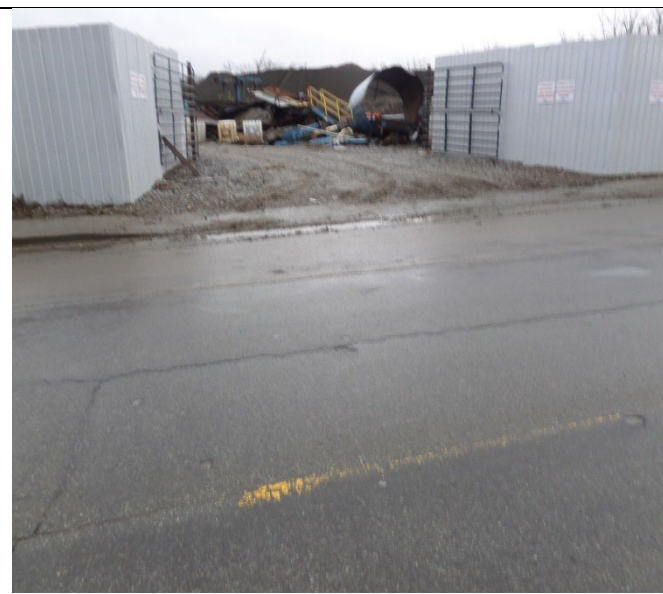
3320 Empire Boulevard. The inspectors observed ASR material on the east side of the road and north down the hill. Photograph 4 taken at 9:30 a.m.
