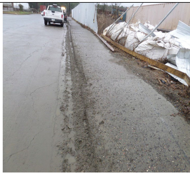
3320 Empire Boulevard. The inspectors observed ASR material on the east side of the road and north down the hill. Photograph 8 taken at 9:30 a.m.
